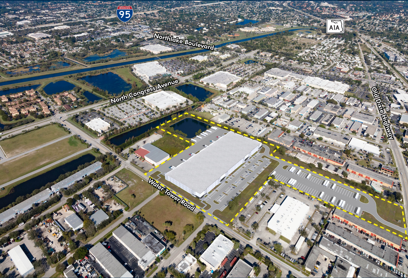
CONSTRUCTION PHOTO- JAN 2023
